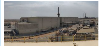
Complete storage and treatment plant for NORM wastes
