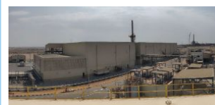
Complete storage and treatment plant for NORM wastes
